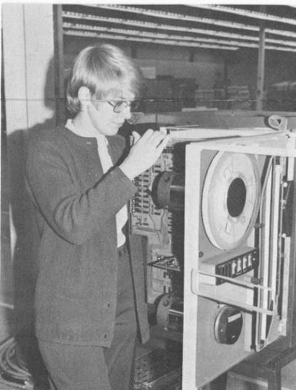
Testing is an integral part of all manufacturing processes at Data General. Lois Stolz inspects just assembled mag tape units.
