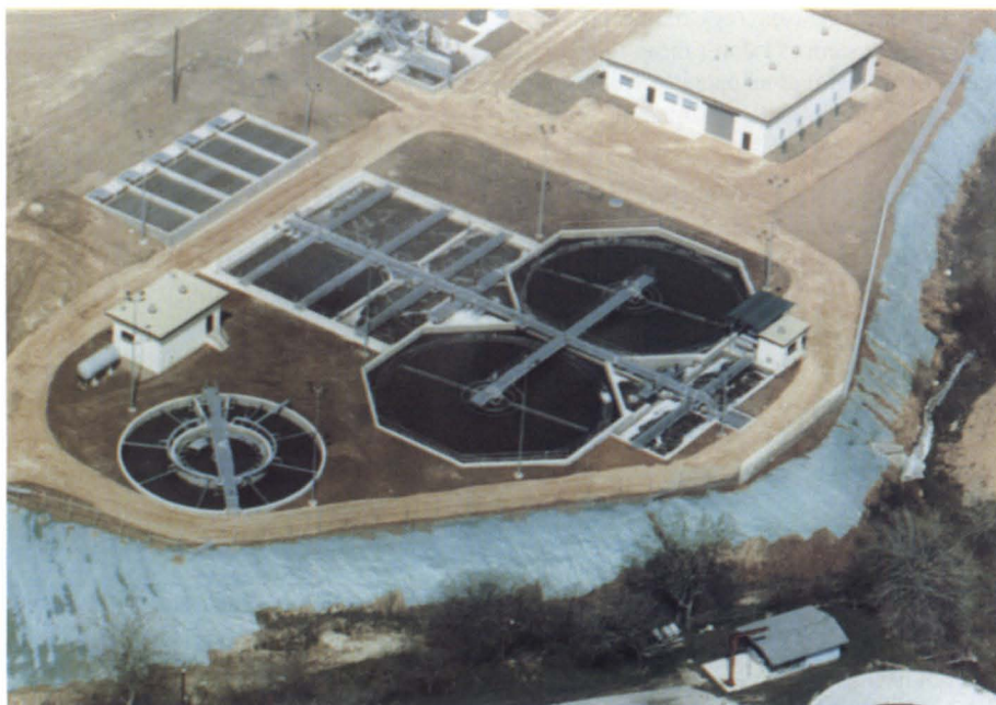
The Kuehler Wastewater Treatment Facility in New Braunfels, Texas, will be using a knowledge-based system to help keep the Guadalupe River clean.
