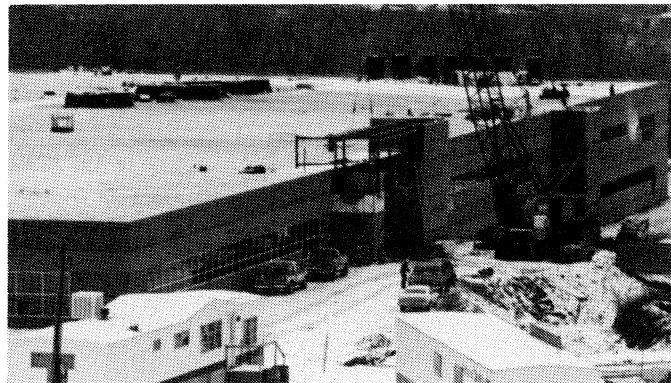
Work progresses on Data General's facility in Fountain.
